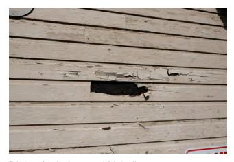
Exterior wall water damage and deterioration
