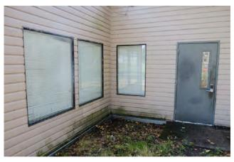
North-east exterior walls with evident ewater damage
