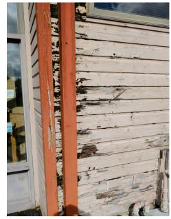
Exterior wall water damage and deterioration
