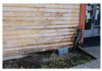
Exterior wall water damage and deterioration
