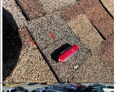
Photograph 64: Cracked shingles at the south sloping roof. (Arrows)
