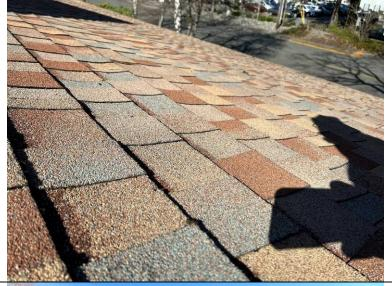
Photograph 25: Slight curling or cupping of the Tamko shingles was observed in various areas of the roof.
