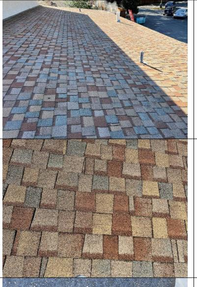
Photograph 22: Looking laterally across the Tamko architectural laminate shingles.
