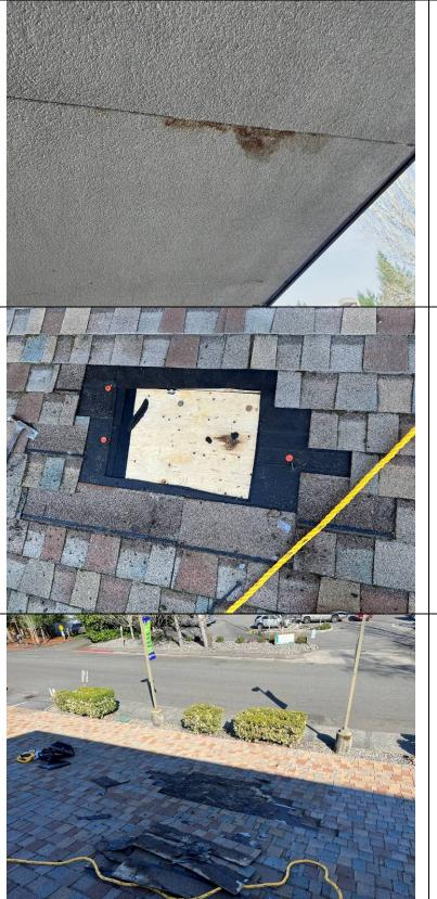
Photograph 7: Water staining at the soffit under the area where test openings were made.
