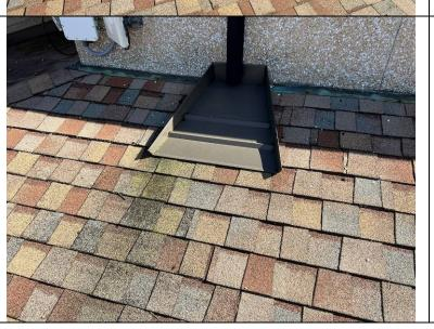
Photograph 66: Splash pad beneath the downspout from the upper roof.
