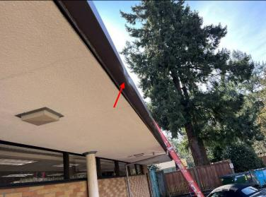
Photograph 68: Damaged gutter (arrow) at the west side of the roof.
