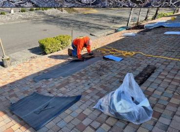
Photograph 21: Temporary roof repairs were made with self-adhered membrane integrated into the shingles in a water shedding manner.
