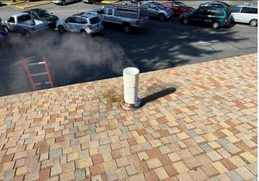
Photograph 65: Boiler vent penetration.
