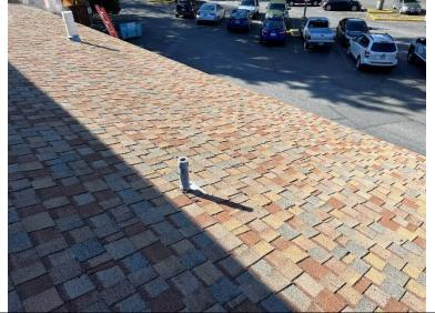
Photograph 34: Typical pipe penetration flashed with a lead penetration flashing.
