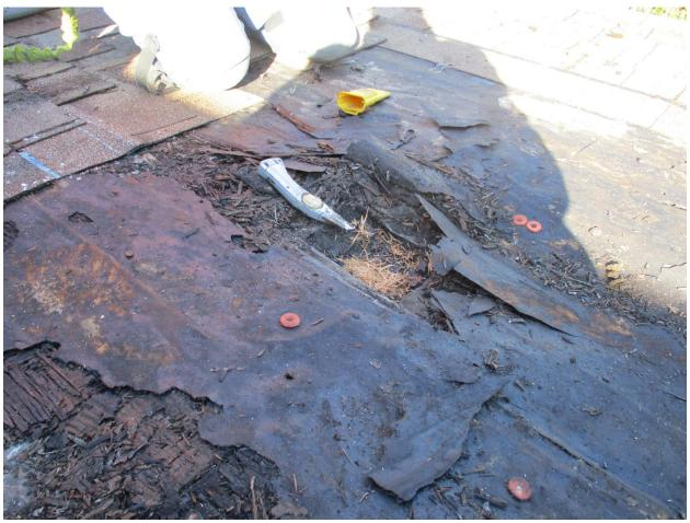
Photo 1 – Deteriorated Plywood Low Roof @ North
