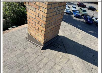
Photograph 93: Closer view of the sheet metal chimney flashing.
