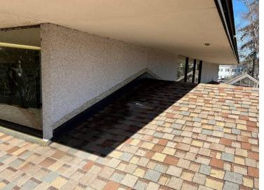
Photograph 32: Roof to wall transition along a rake wall.
