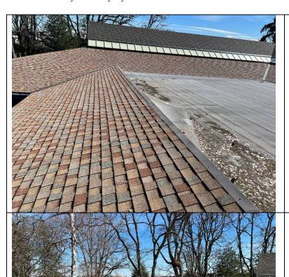
Photograph 43: Steep slope to low slope roof transition.
