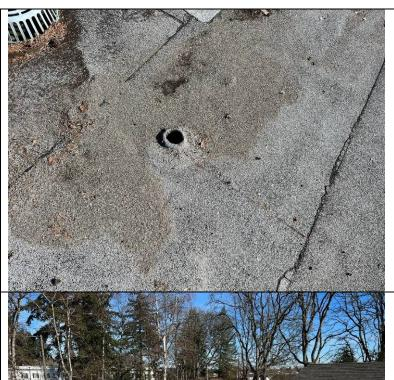
Photograph 76: Closer view of the contractor style overflow.
