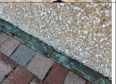
Photograph 33: Closer view of the headwall flashing.
