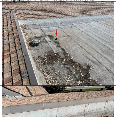
Photograph 74: Typical cast iron roof drain and adjacent contractor style overflow (arrow).
