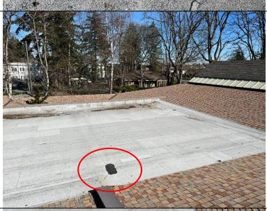
Photograph 77: Roof cement patch over an apparent location of damage.
