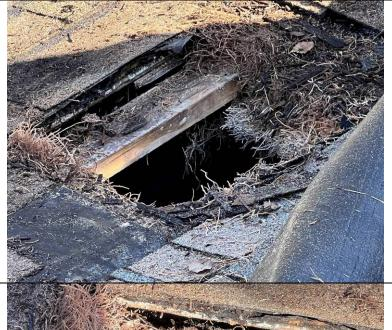
Photograph 19: Closer view of test opening #4 showing the deteriorated cementitious wood fiber substrate board.
