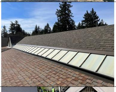
Photograph 41: Low roof to high roof transition at the translucent skylight panels.
