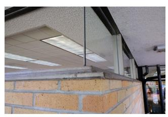
Single pane windows with failed seal at corner joint
