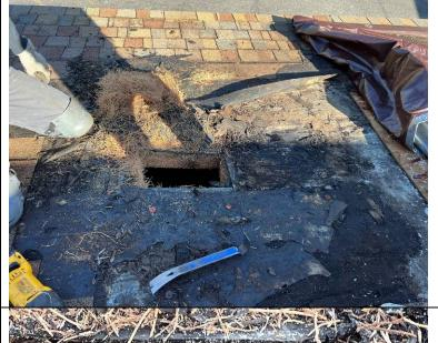
Photograph 13: Portion of the cementitious wood fiber substrate was removed to provide visual access to the structure below.
