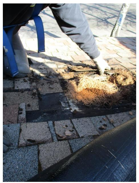
**Photo 3 - Tectum Water Damage**
