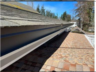
Photograph 101: Eave edge without a gutter.
