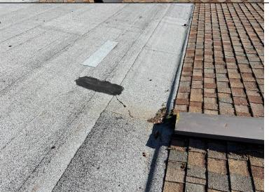
Photograph 78: Closer view of the roof cement patch circled in Photograph 77.
