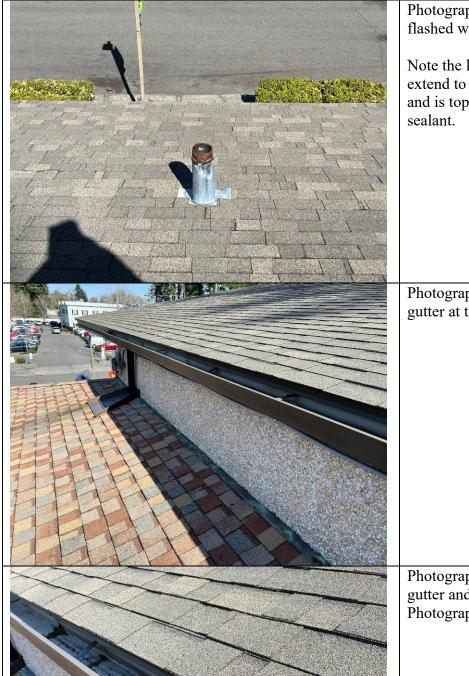
Photograph 97: Pipe penetration flashed with a lead flashing.
