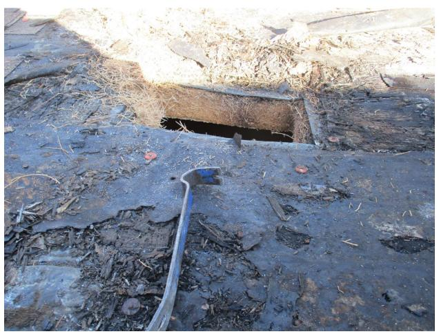
Photo 2 – Tectum Structural Panel Section
