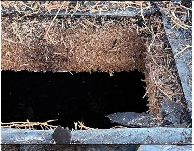
Photograph 14: Closer view of the cementitious wood fiber substrate board at the test opening.
